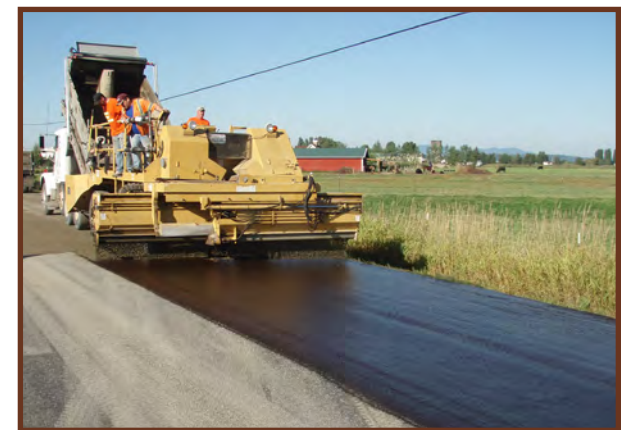
Roadway Resurfacing in Skagit County
