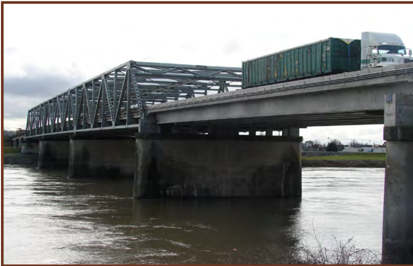
Interstate 5 Bridge over Skagit
