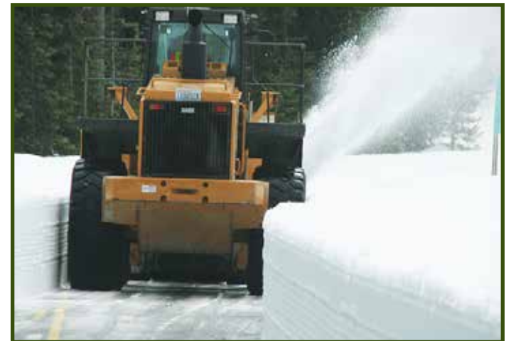
Roadway Maintenance on State Route 20
