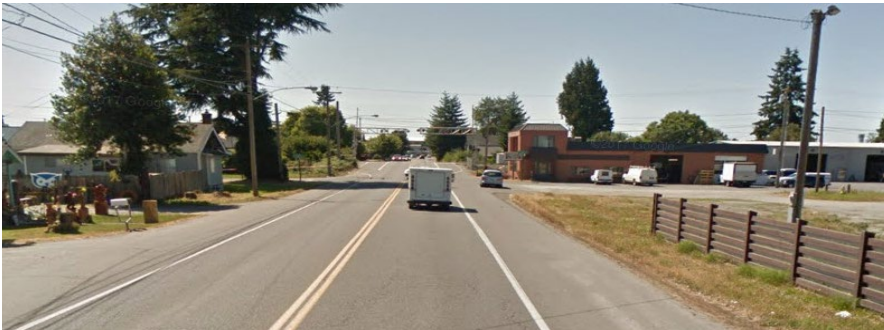
Current Conditions at SR 20 (Alder St to Cascade Hwy)
