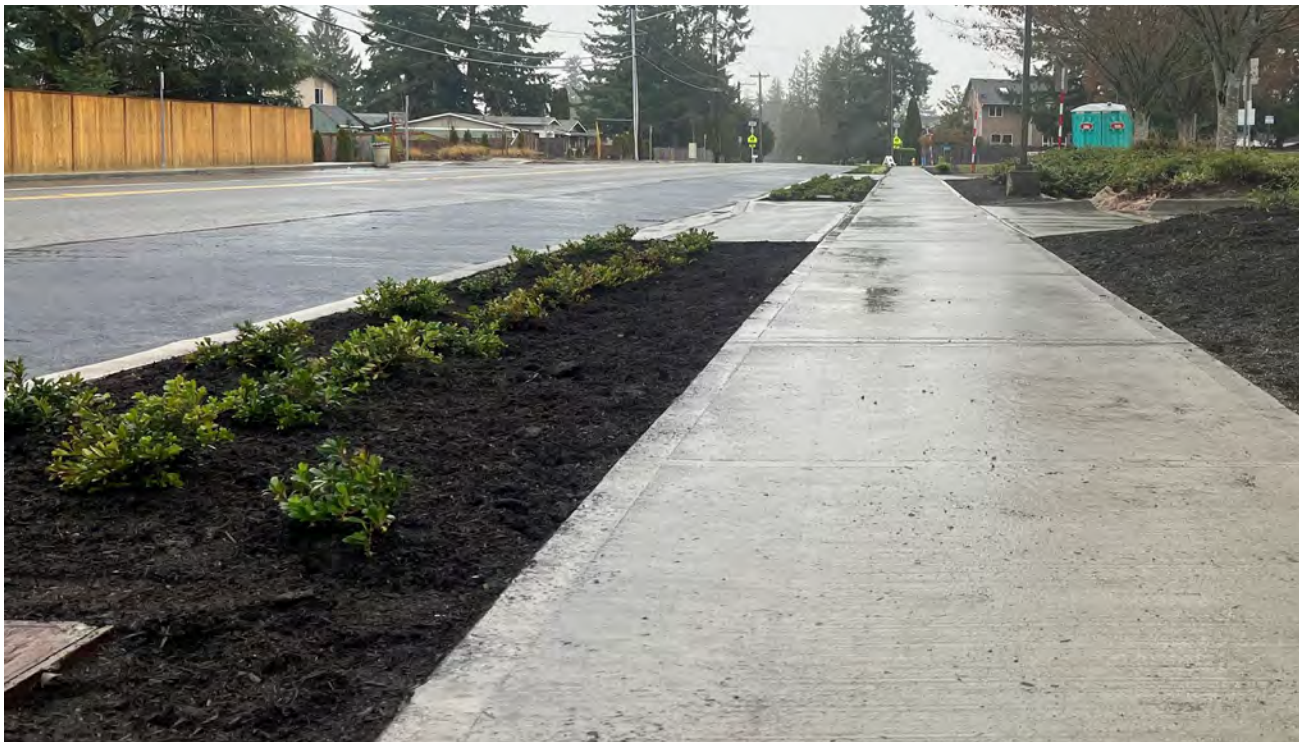
Sidewalk in Snohomish County. Photo Credit: Snohomish County.
